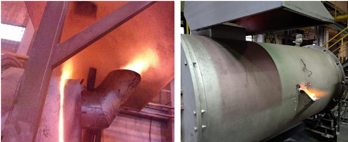
Figure 1. Blasting of emissions through openings
