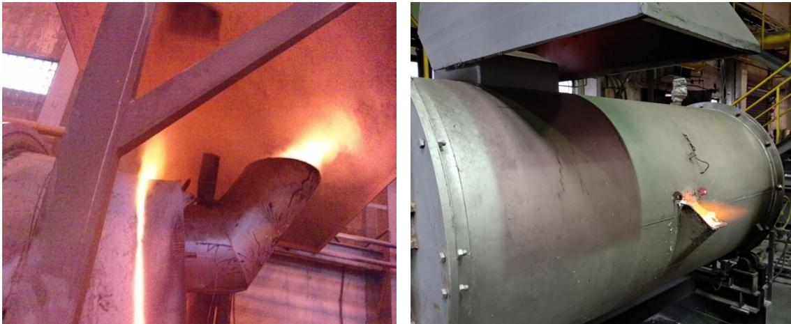
Figure 1. Blasting of emissions through openings
